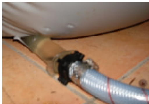
LIFT SIDE OF POOL TO CHECK THAT THIS TUBE FITTING IS NOT CRUSHED UNDER THE POOL AND THAT WATER FLOWS FREELY ESPECIALLY CHECK INSIDE THE POOL WHERE IT ENTERS.
